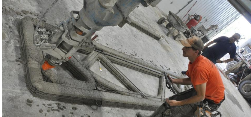
Figure 4. Partial printing and reinforcing of the last layer
