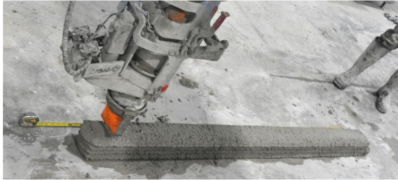
Figure 2. Process of printing the fourth layer of the beams
