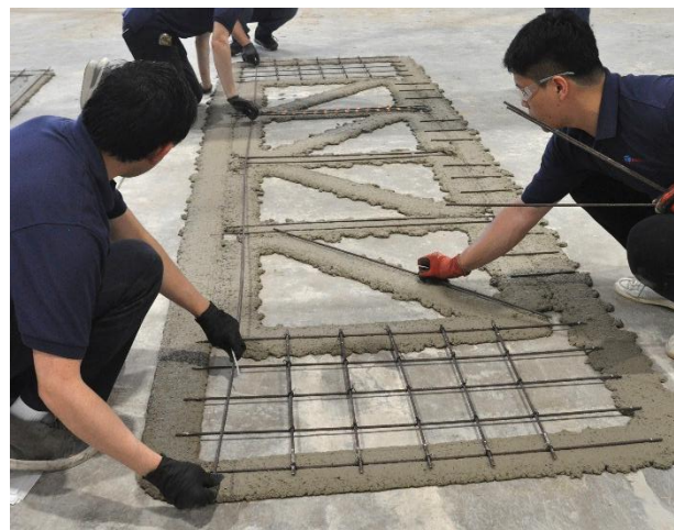
Figure 3. Insertion of reinforcement
