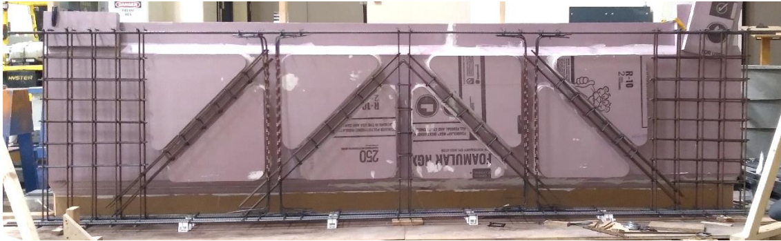
Figure 4. Precast trussed web girder formwork and steel
