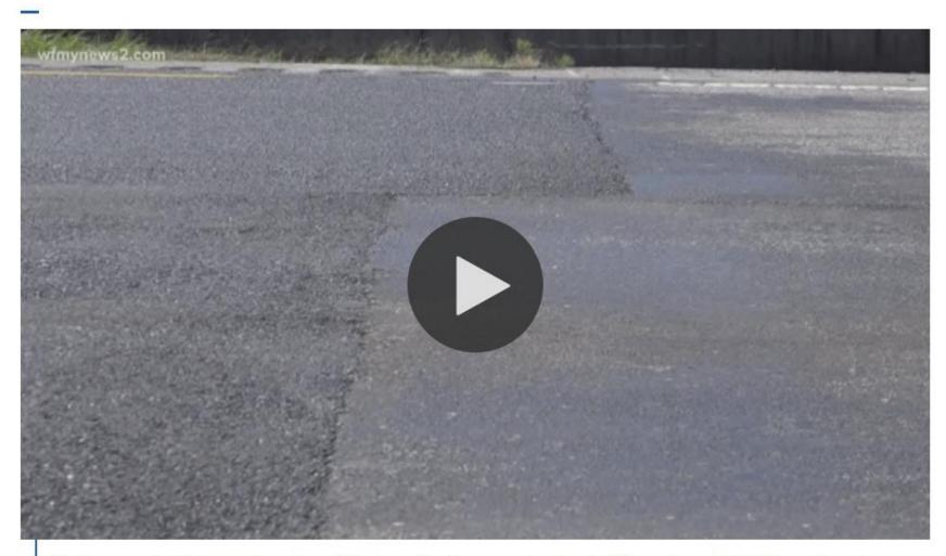
That new project is happening along I-85 where it spits as you head out of Greensboro. NCDOT is putting down a new layer of asphalt to make the roads safer when it rains.
