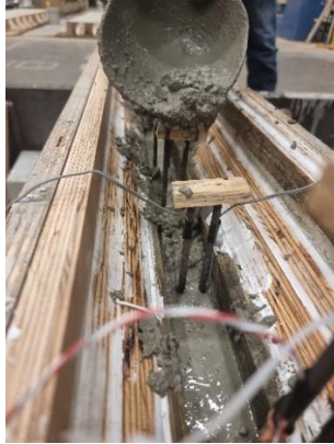
(c) Concrete casting
