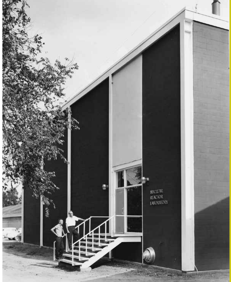
Former Nuclear Reactor Building on campus
