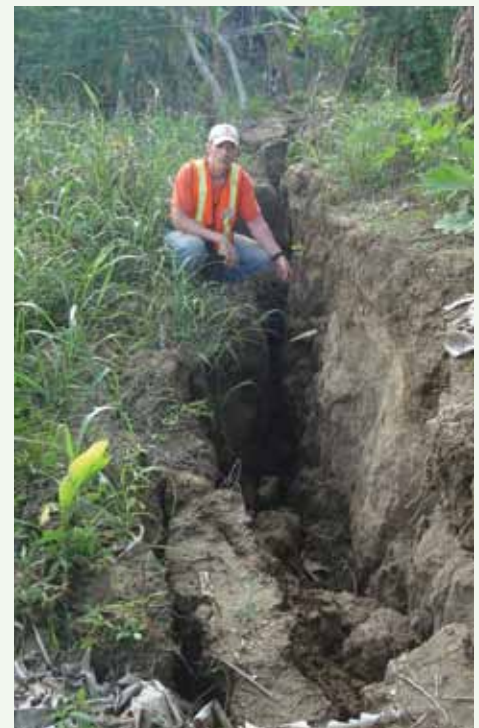
On his second trip to Haiti, Associate Professor Scott Olson examines a failed slope.
