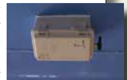
A box containing one of many wireless smart sensors, affixed to the Jindo Bridge.
