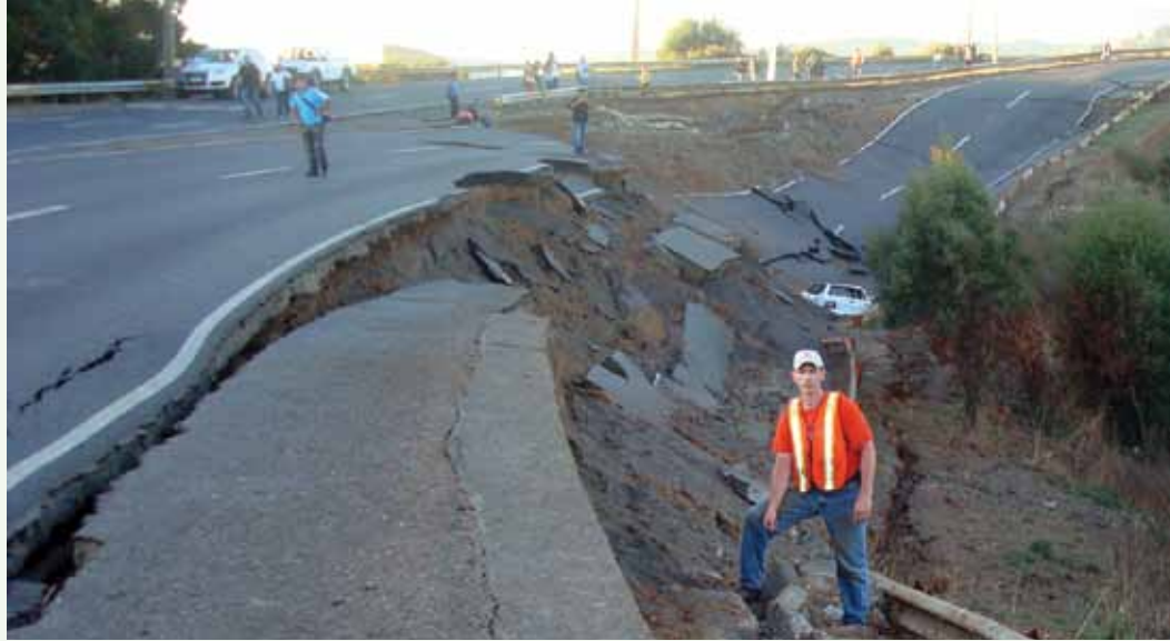
Associate Professor Scott Olson examines a failed highway bridge on a study trip to Chile.
