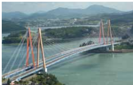
The Jindo Bridge in South Korea, on which the wireless monitoring is currently deployed.
