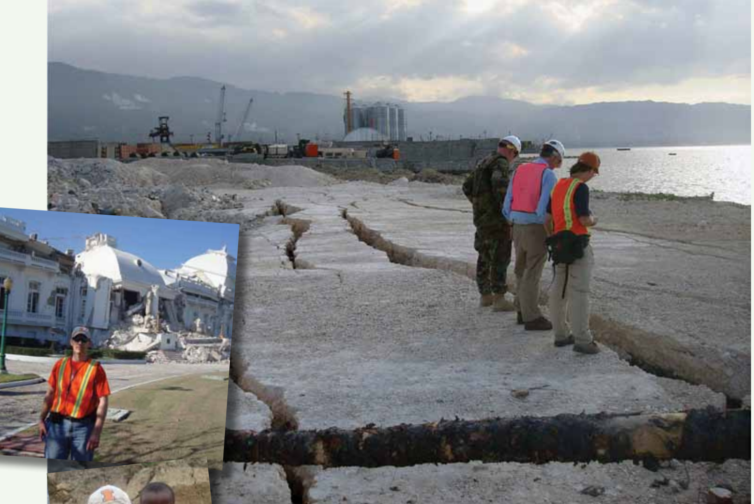
▲ Engineers examine the damage to the port in Port-au-Prince, Haiti. Top left: Associate Professor Scott Olson stands before the destroyed Presidential Palace during his first visit to Haiti. Bottom left: A Haitian girl tries on Olson's signature Illinois hat.
