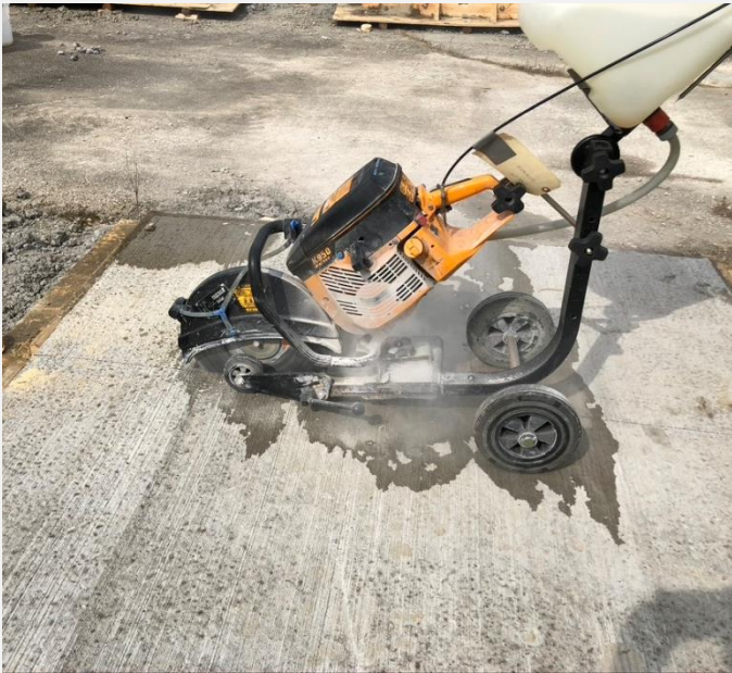
Saw Cut 6-in-deep
