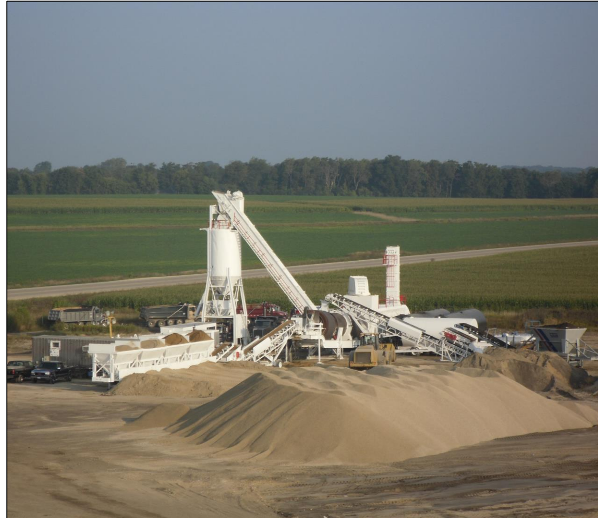
Photo courtesy of Rock Road Companies, Inc.
