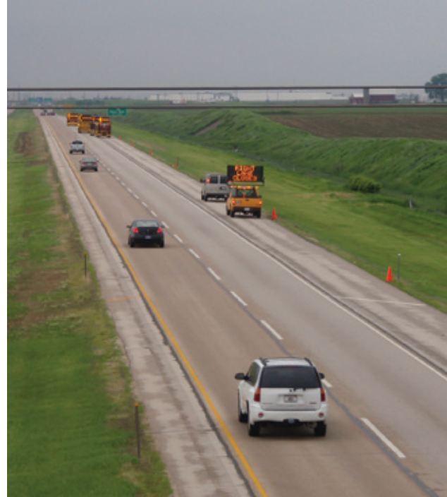
A rolling lane closure moves through an interstate work zone.
