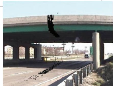
Scan of damaged bridge girders on Illinois Route 162 bridge over I-55/70, Troy, Illinois.
