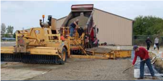
A full-scale test section is constructed at ATREL.
