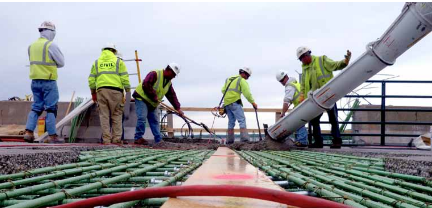
Above: Repairs on the structure that carries I-80 over the Mississippi River. Photos courtesy of IDOT District 2 contractor Civil Constructors, Inc.
