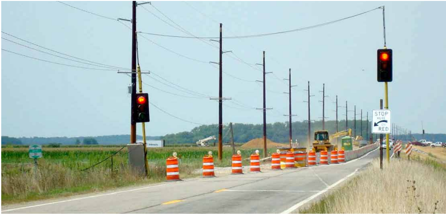
Above: Traffic control provided during structure replacement on IL 15 near the Edwards County line. Photo courtesy of IDOT District 7 contractor E.T. Simonds Construction Company.
