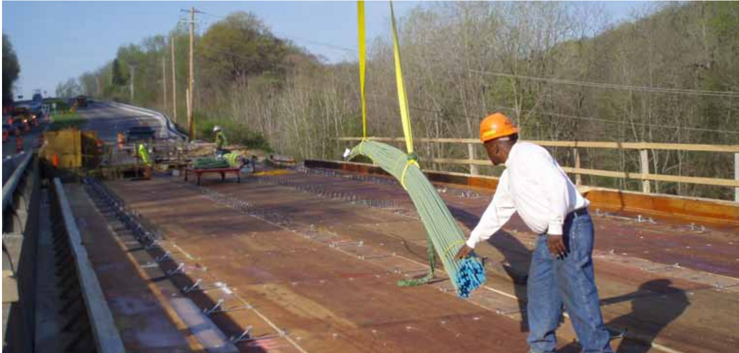
Below: Installation of all epoxy reinforcement bars and tie bars in the superstructure on Airport Road in Peoria County. Photo courtesy of IDOT District 4 contractors R. A. Cullinan & Son, a division of UCM, Inc., and Central Illinois Rebar Installers, Inc.
