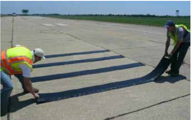
Temporary rumble strips were installed so researchers could study how well they generated sound levels to enhance the alertness of drive-by motorists.
