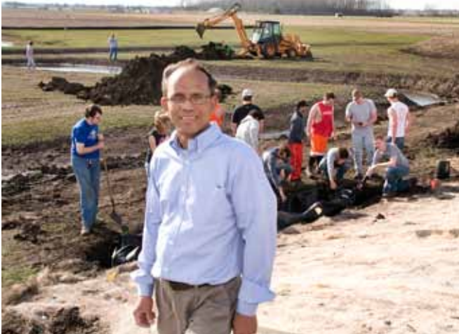
Co-PI Prasanta Kalita stands in front of construction for the ICT's erosion control center.
