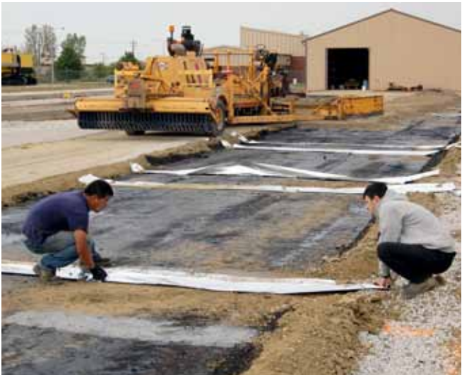
Students help construct a test pavement at ATREL.
