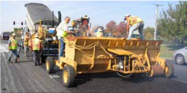
A quartzite sprinkle treatment is added to the test pavement.
