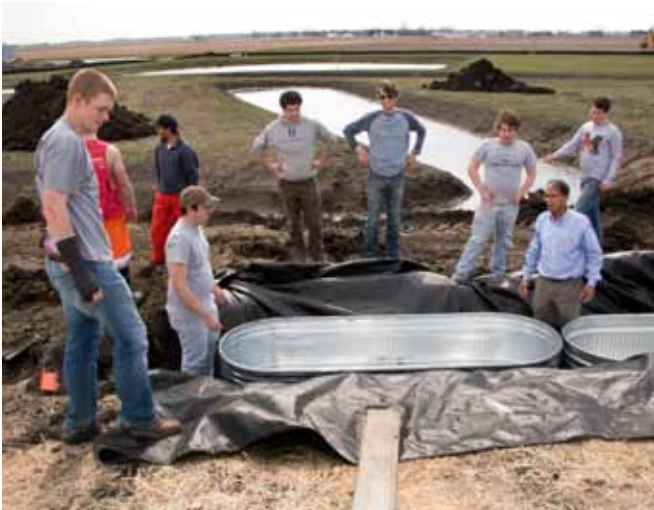
Installation of runoff and sediment collection tanks.
