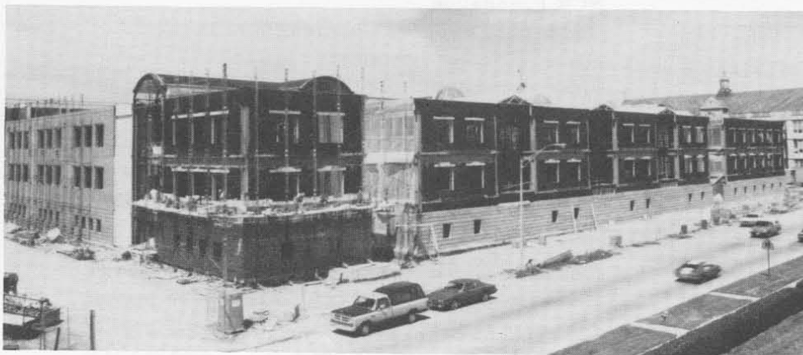
June 16, 1989. Looking northeast, the brick exterior is being laid.
