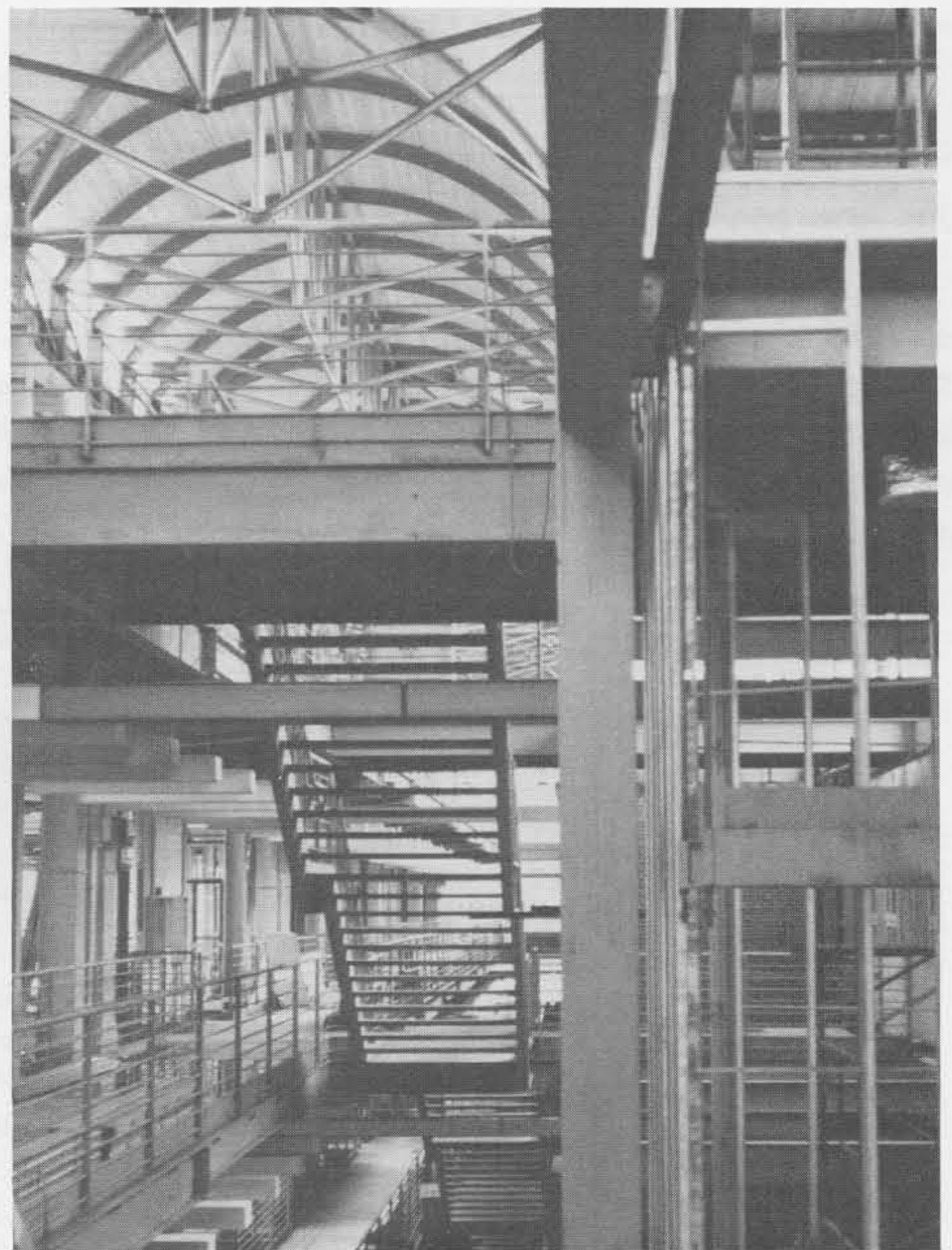
March 18, 1989. Looking west, along the second floor corridor.
