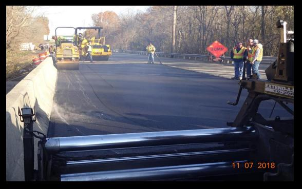
Application of 9.5 FG surface course. Paver without auger extensions.
