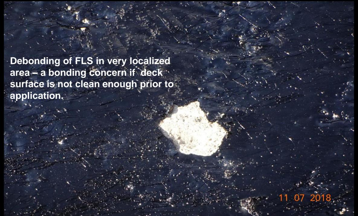
Debonding of FLS in very localized area – a bonding concern if deck surface is not clean enough prior to application.
