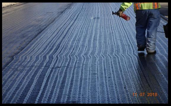
Application of 9.5 FG surface course. Paver without auger extensions.
