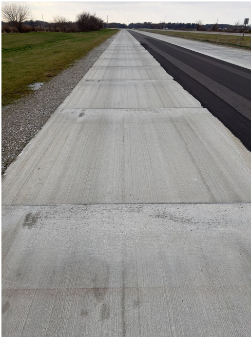
Artificial Faulting Section
