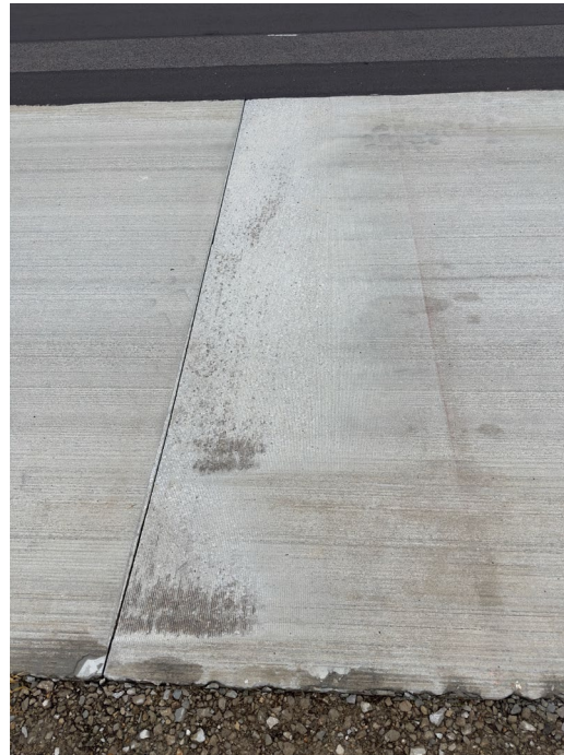
Faulted Joint
