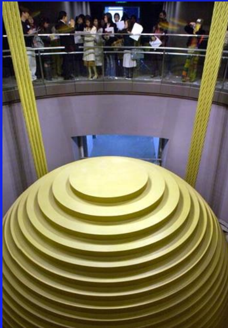
Tuned mass damper (pendulum) in Taipei 101
