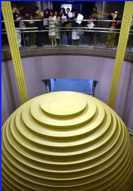
Tuned mass damper (pendulum) in Taipei 101
