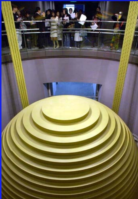
Tuned mass damper (pendulum) in Taipei 101
