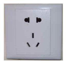
Appliances such as hair dryers, irons, blenders, etc. rarely have international ratings and most likely are not safe to operate on 220 V unless purchased in China. Transformers to step down 220 V to 110 V can be bought online in the US and China, but the frequency is 50 Hz so this is not a universal solution. Always check before plugging in any US appliance or electronic into a Chinese outlet for the voltage input rating, since 120 V devices will be damaged or destroyed by 220 V power.
