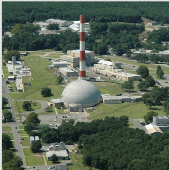
The High Flux Beam Reactor (HFBR) at Brookhaven National Laboratory
