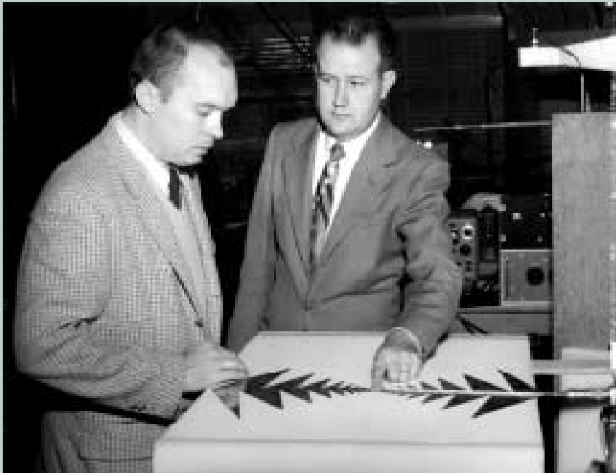
Dwight Isbell (left) and Paul Mayes discuss the feed point of a planar, log-periodic, triangular toothed array (c. 1957).
