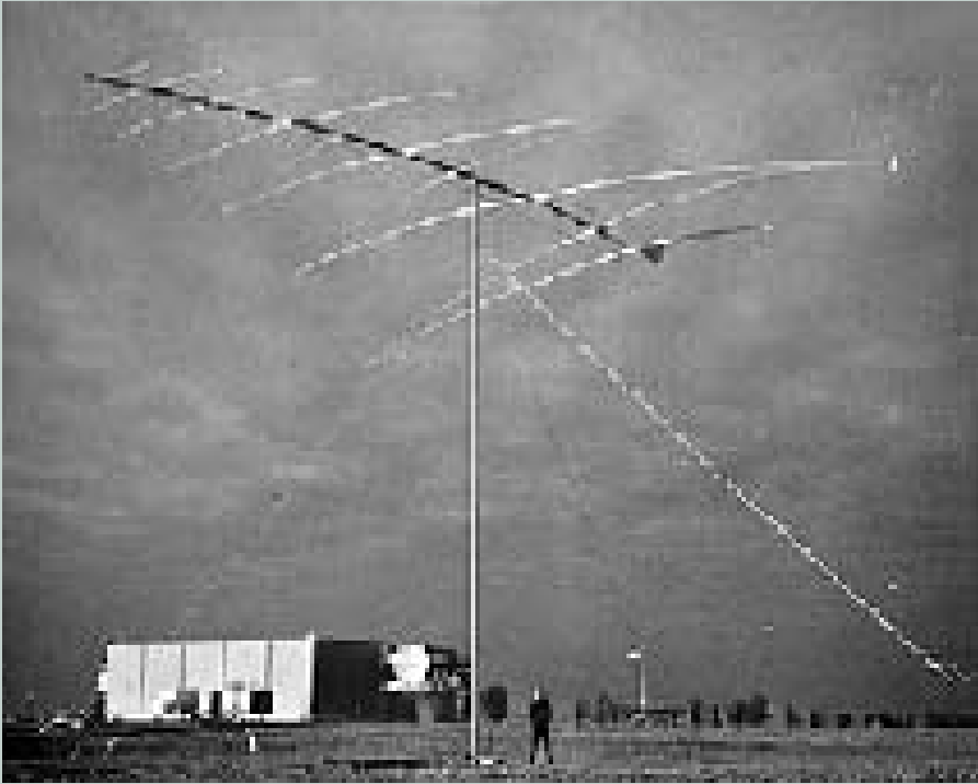
Early commercial version of a wire outline, log-periodic, triangular toothed array.
