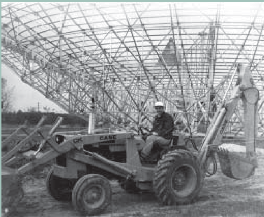
Doing engineering the old fashioned way. George Swenson helps with construction of the 120-foot telescope.
