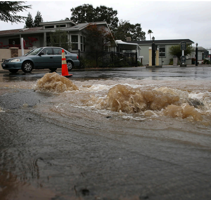
A water main break following a 6.0 earthquake in Napa, California.
