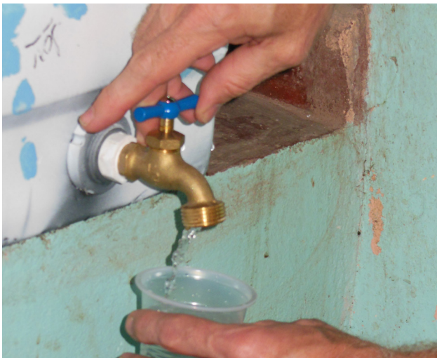
A team member opens the valve to get the first cup of clean water from the system.
