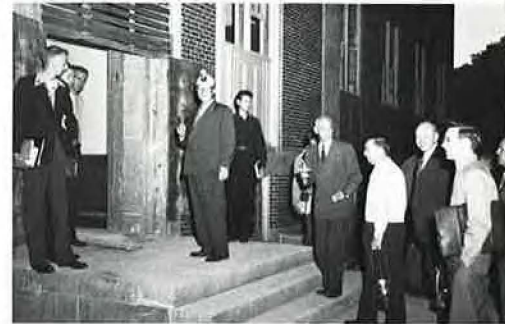
Entering the newly completed building, now known as Everitt Laboratory.
