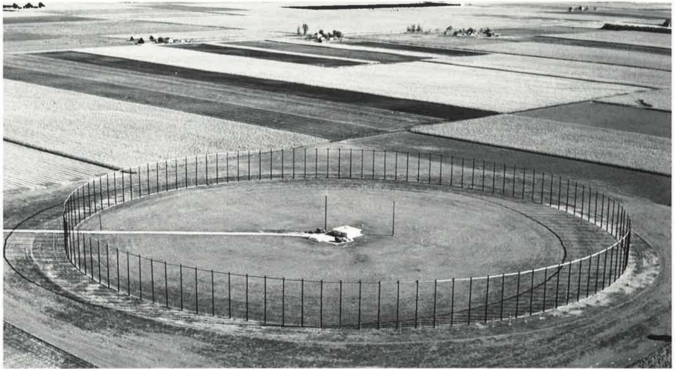
A large-aperture radio direction finding system known as a Wullenweber array at the Bondville Road Field Station, October 1960. Operating at a frequency range from 4 to 16 MHz, the array uses 120 antennas and is 1000 ft in diameter.
