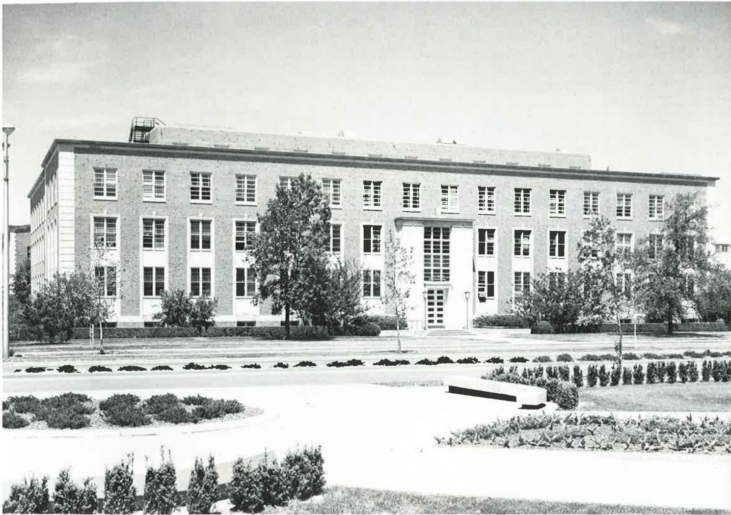
Dedicated in 1949, the Electrical Engineering Building was later renamed the William L. Everitt Laboratory. The third floor was added in 1965.
