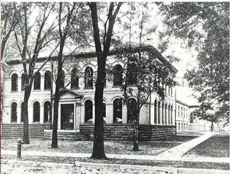
Applied Mechanics Laboratory in 1928. This space was assigned to electrical engineering when a new building (later renamed Talbot Laboratory) was constructed for the Department of Theoretical and Applied Mechanics.
