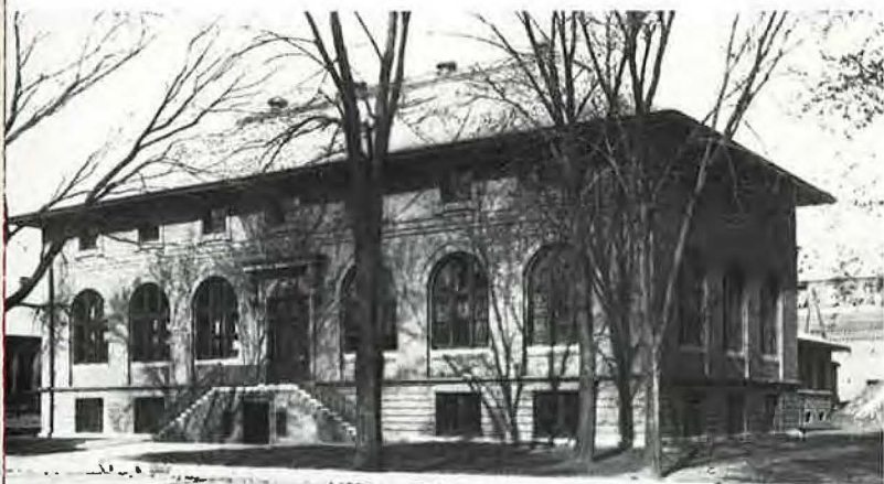
The Mechanical and Electrical Engineering Building in the early 1900–05 era. Note the boiler house for the Boneyard Power Plant in the right background.
