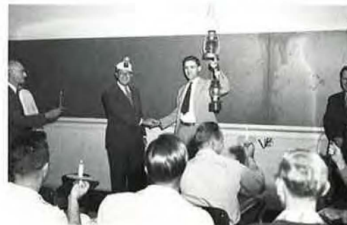
"Newly completed except for the electricity!" The first class was held using candles and miners helmets for illumination.
