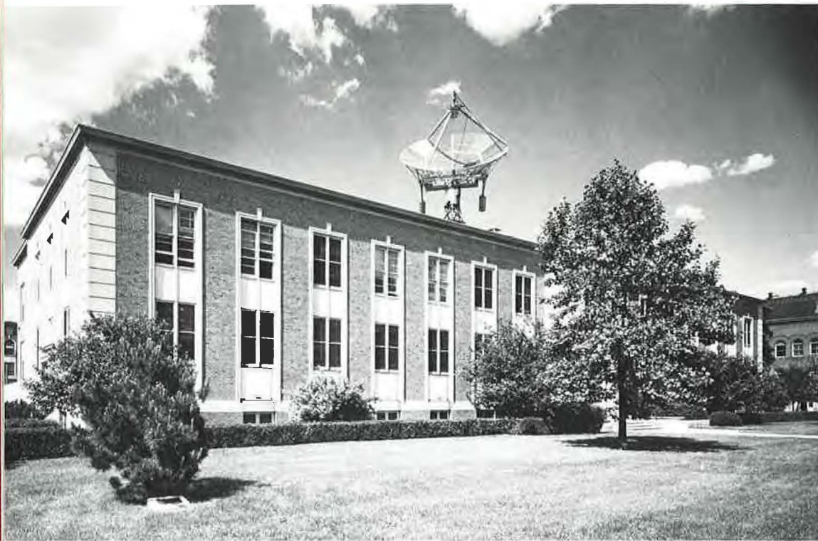
The Electrical Engineering Building (renamed Everitt Laboratory) before the addition of the top floor. In 1958, a unidirectional antenna was installed on the roof as a feed on a "moon-bounce" parabolic reflector. This was the first application of a log periodic antenna.
