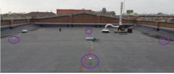
Fig. 4: Four antennas located on roof of Talbot Laboratory, University of Illinois at Urbana-Champaign. Reference image of the setup taken from [7]
