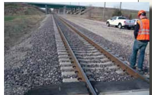
Lecturer J. Riley Edwards inspects closely spaced concrete ties at a recently upgraded UP crossing near Springfield, Ill.
