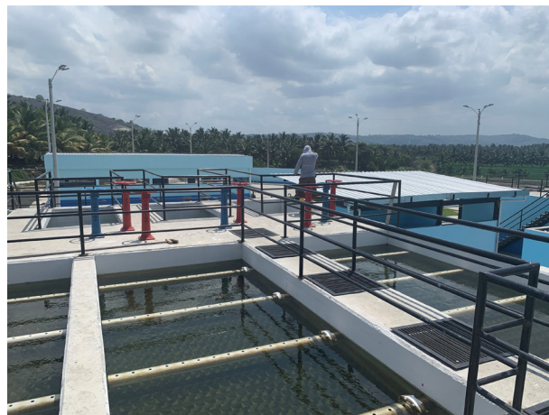
Rocafuerte, the municipal water supply nearest to El Guarango, Ecuador, features a new surface water treatment plant with polymer coagulation, filtration, and chlorination.
