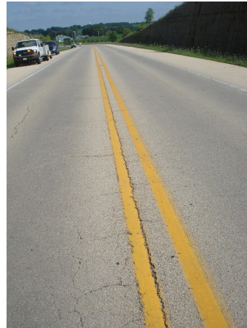
Route 26 with Joint Sealant
