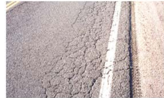
Fatigue Cracking
