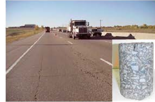
Top-down Cracking
