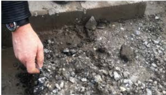
Moisture Damage
