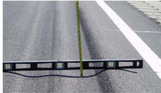
Permanent Deformation
