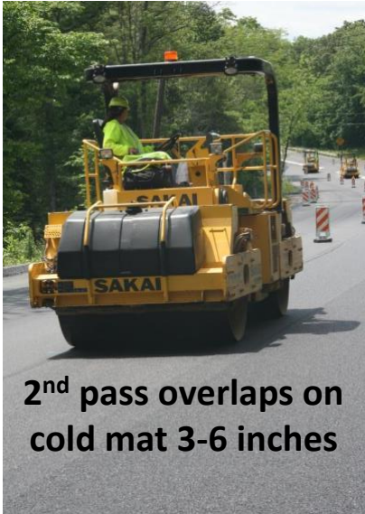
1 st pass all on hot mat with roller edge off joint approx 6-12 inches
