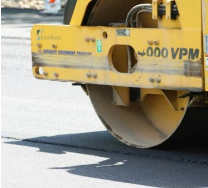
1 st pass all on hot mat with roller edge off joint approx 6-12 inches
