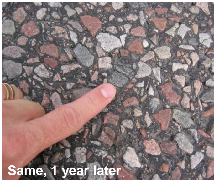
New SMA pavement
