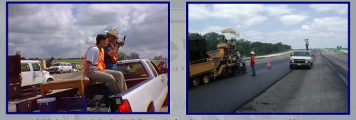
Initial research included the use of a thermal camera operated by a researcher in the back of a pickup truck. In addition to obvious safety considerations, this initial method was found not to be practical. A series of infrared images had to be manually combined to produce a complete profile. Distance and position data were also difficult to incorporate.
