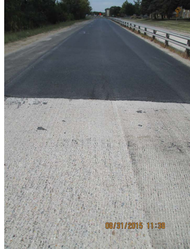
2015 UBWC atop PCCP Fine Mill
