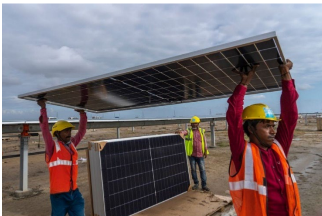
Installing solar panels at Adani Green Energy's Renewable Energy Park in India. Photo: Rafiq Maqbool/Associated Press
