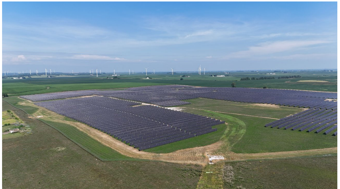
Aerial image of the first stage of Earthrise Energy's 270 MW e solar farm, which will eventually house more than 595,000 bifacial solar modules of 590 W each, and 75 4-MW e inverters. Image credit: Earthrise Energy
