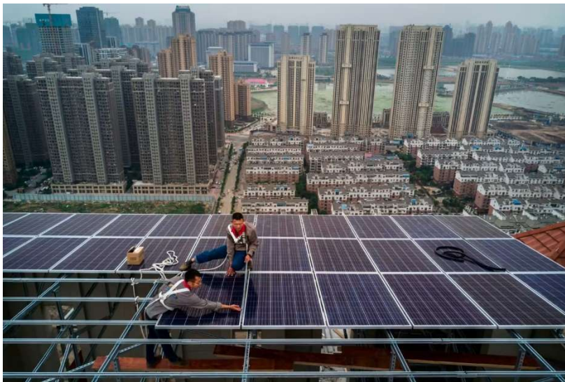
Workers install solar panels in Wuhan, China. Buoyed by massive domestic demand, Chinese manufacturing of polysilicon and its processing results in a product that is two-thirds the price of a European-made product. Image credit: Financial Times.
