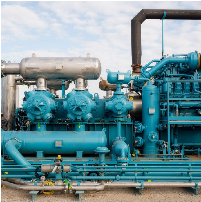
BKV compressor units process carbon dioxide in Bridgeport, Texas, before it is injected into a well. Denver-based BKV says that by the 2030s it will store millions of tons of climate-warming carbon dioxide in wells deep underground to eliminate or offset all the emissions generated from manufacturing and using its gas. Image credit: The Wall Street Journal.
