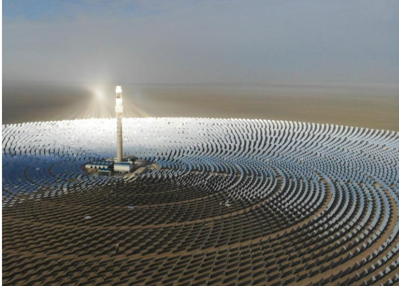
A recently completed 100-MW concentrated solar power plant located in Dunhuang, northwest China's Gansu Province. The plant uses 12,000 mirrors that concentrate the sunlight onto a receiver at the top of a solar tower, which then heats molten salt. The molten salt exchanges heat with water, to produce steam that drives turbines. The plant is designed to generate 390 million kWh of power annually, which can reduce carbon dioxide emissions by 350,000 metric tons per year, compared to a similarly sized natural gas-fired steam power plant. Image credit: www.xinhuanet.com
