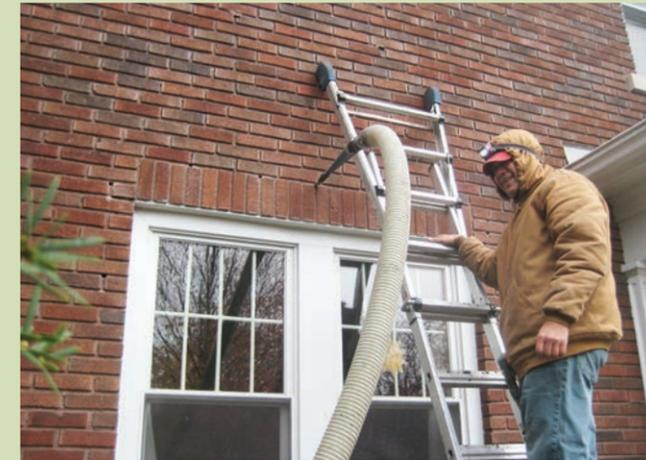
Blowing dense-pack cellulose into the wall cavity through 1-inch holes in the mortar joints from the exterior. The work is barely visible afterwards.
