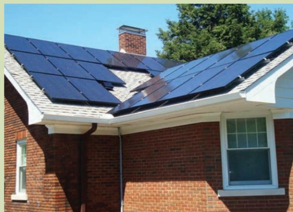
The solar photovoltaic array on the house. Most of the modules face south, with some west-facing modules shown on the addition. The tree is a mature Japanese maple, which is not tall enough to shade the modules.
