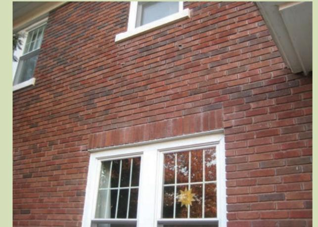
through the mortar joints and patiently blew in the cellulose from the exterior. He did not touch any interior walls. He then insulated and sealed the rim joist in the basement using closed-cell foam (R-13). Finally, he added weather stripping to the exterior doors and attached a 2-inch foam board to the back of the attic door.
