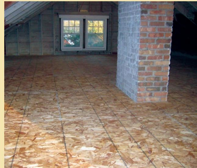
(left) The attic floor prior to the second round of weatherization. In the first round, done many years earlier, 5 ½ inches of cellulose were blown under the floorboards, and the ductwork was wrapped in fiberglass insulation. (right) The attic after the second round of weatherization. A frame was built from 2 x 10s to contain 9 inches of loose pack cellulose, after which a plywood floor was added.
