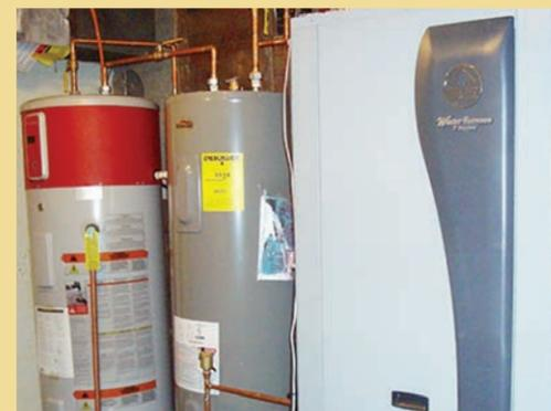
The ground-source heat pump is on the right, the air-source heat pump water heater is on the left, and the storage tank is in the middle. There is plumbing to draw water from the bottom of the storage tank in the summer and use it to cool the ground-source heat pump before returning the water to the top of the storage tank. The water heater draws this preheated water from the storage tank as needed.
